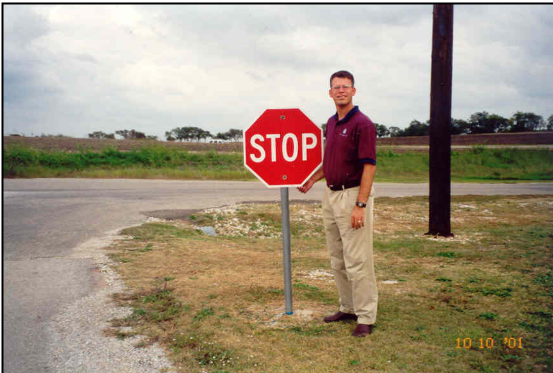
Figure 49. Sign on Elementary Site Mounted Several Feet below the Standard Height.
