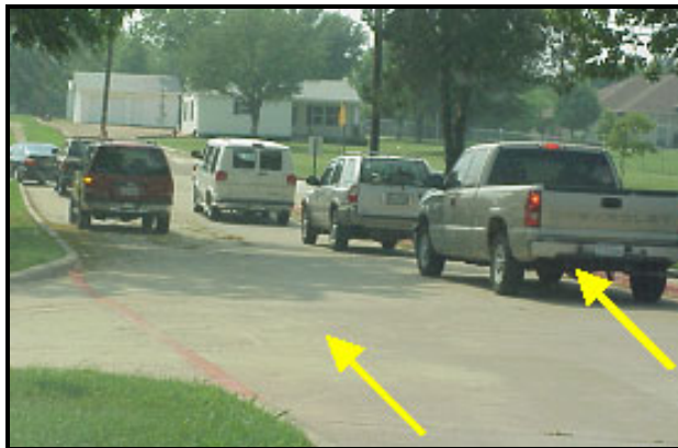
Figure 44. School Exit Driveway with Two Lanes for Left and Right Turn Movements.
