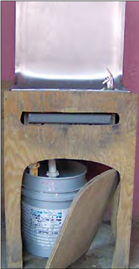
Water efficiency is a key element of sustainable design, sorely lacking in this Virgin Islands school.
