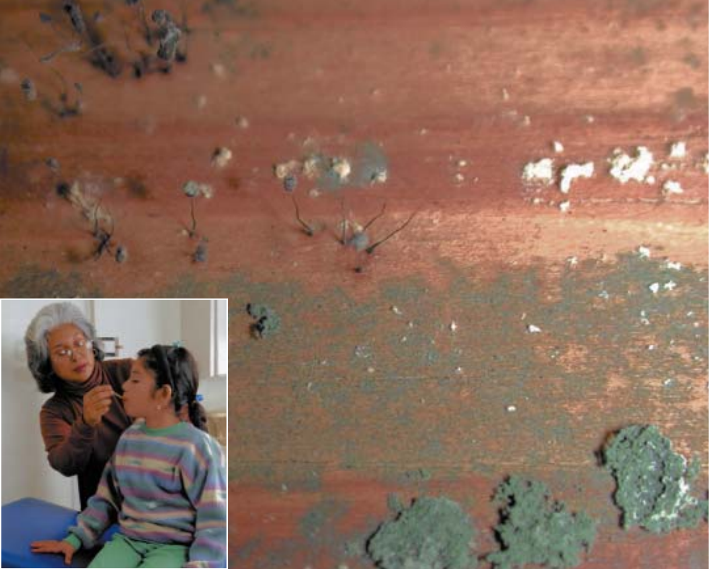
Mold on joist, photo by Daniel Friedman
