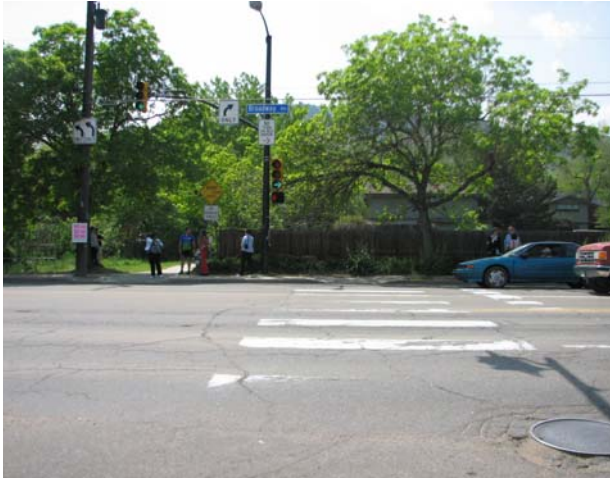
Worn signs, crosswalk markings, and other markings should be replaced.
