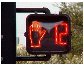
Pedestrian countdown signals provide pedestrians with information about time remaining in the crossing phase. (photo: Oakland Metropolitan Transportation Commission)
