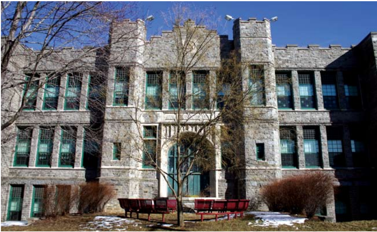
Although the original entrance to the Media Elementary School, top, is no longer used, it remains an integral part of the historic integrity of the school, parts of which were built in 1915, 1929 and 1951. The main entrance was moved to the side during major renovations in 1994.
