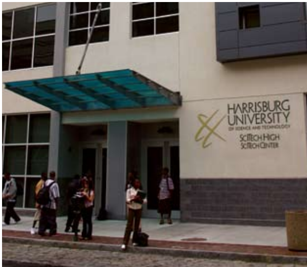
ABOVE: The Harrisburg School District's new SciTech High School, serving 500 students in downtown Harrisburg, was created by renovating and adaptively reusing the former Harrisburg YWCA, which itself was created by combining and renovating three stores.
