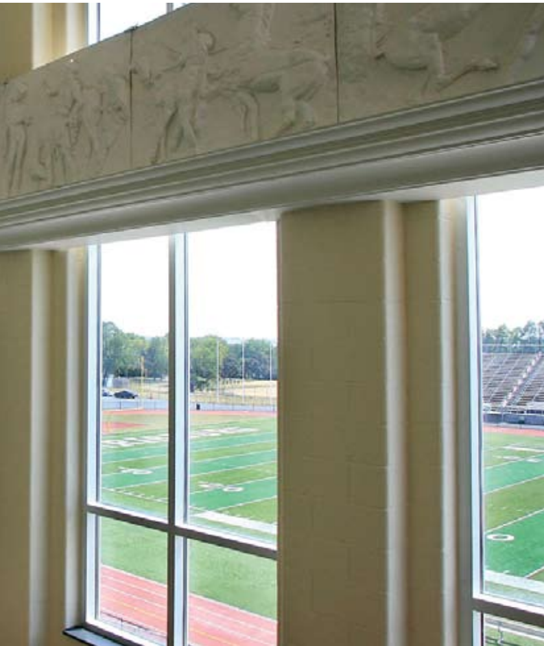
copy the original building in two phases during the renovation process, which will be completed in September 2007. Above, the new library, which includes marble carvings from the original structure, overlooks the football field.
