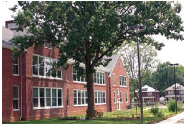
The 1936 Schaeffer Elementary School was renovated and enlarged in 2002.
