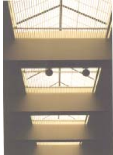
Linear skylight in multipurpose room includes electrically operated louvers to reduce brightness when needed.
