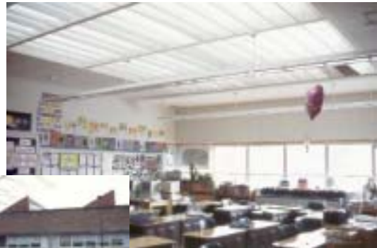
Central sawtooth monitor provides even illumination across desktops in this classroom. NREL/PIX 11406
