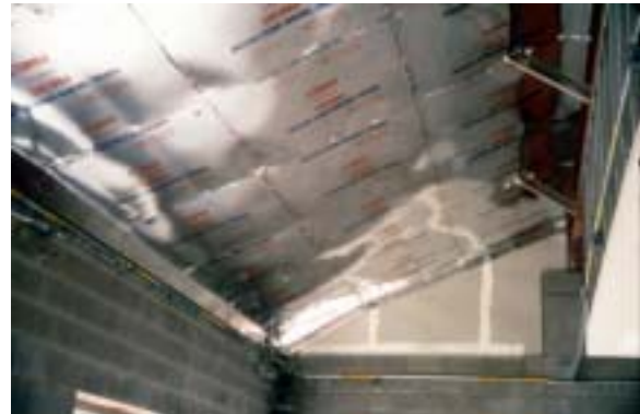
Radiant barriers are recommended for hot and coastal climates, over spaces cooled by air conditioners or natural ventilation. NREL/PIX 11331
