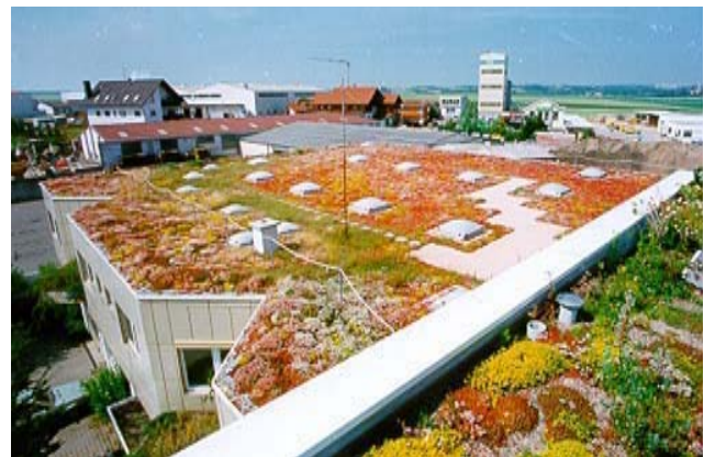
A vegetated roof reduces the amount of rainwater runoff while simultaneously minimizing heat build-up and providing insulation.
