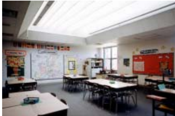
Toplighting reduces the glare and allows for a more even distribution of daylight within a space. NREL/PIX08834
