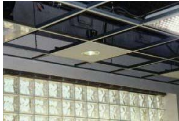
Formaldehyde-free acoustical panels with recycled content are considered a material efficient, low-volatile organic compound product, promoting healthy indoor air.
