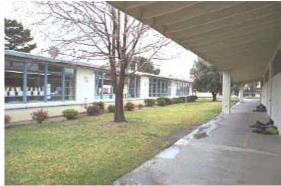
North versus south windows-south windows are shaded from direct sun-but receive daylight reflected off of concrete walk and white painted overhangs. North windows are large and unshaded.
