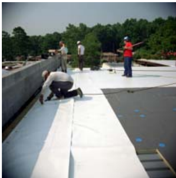
Because solar gain on roofs is a significant component of heat gain, using materials that have a high reflectance can significantly reduce the load. NREL/PIX 03510
