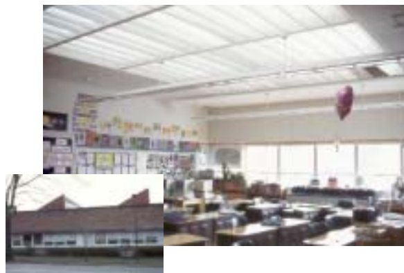
Guideline DL5: Central Toplighting from a sawtooth monitor with sun baffles is combined with DL1: View Windows to provide balanced illumination in a classroom. NREL/PIX 11406
