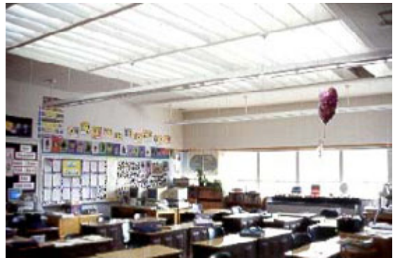
Gentle, diffuse daylight permeates a classroom with both sidelight and toplight. Note that all surfaces are painted white to distribute light more efficiently and reduce contrast glare. NREL/PIX 11392
