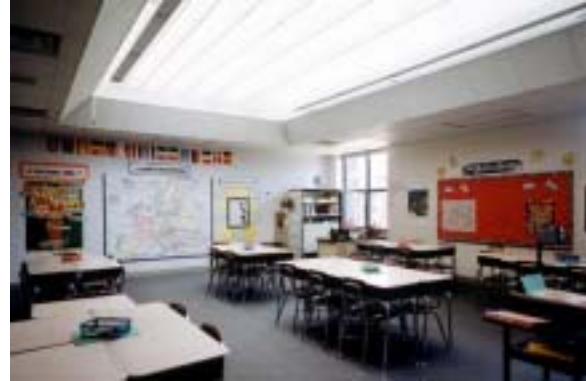
Toplighting reduces glare and allows for a more even distribution of daylight within a space. NREL/PIX 08834
