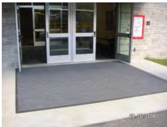
Walk off system at New Hampshire school
