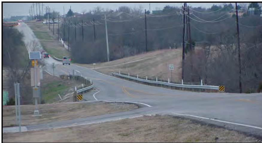
Figure 34. School Site Located on Two-Lane High-Speed Roadway – No Sidewalks.
