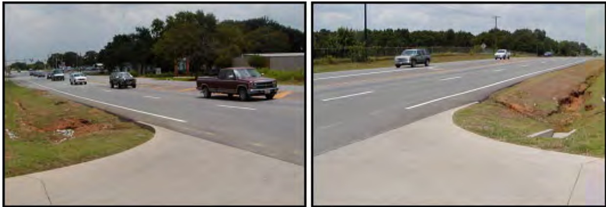
Figure 7. Good Example of School Driveway with Good Sight Distance in Both Directions.
