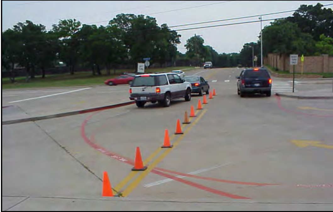
Figure 29. Traffic Cones Placed to Reinforce Turn Restrictions from Exit Driveway.
