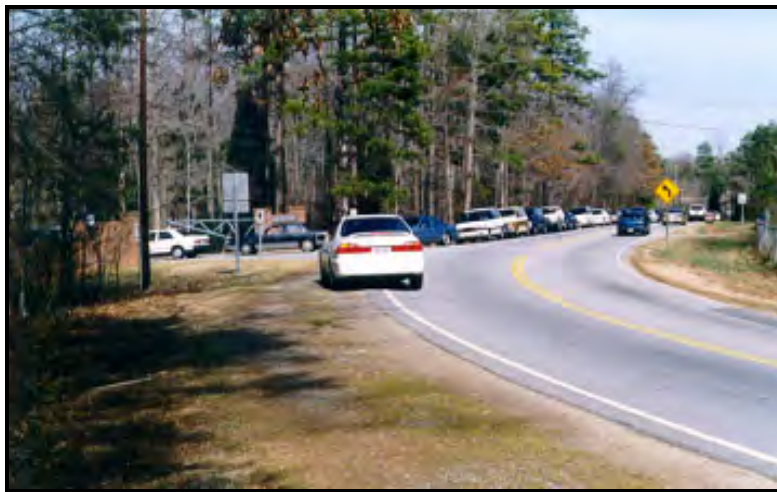
Figure 45. Traffic Queue on Unpaved Shoulder – Right-Turn Lane Might Be Warranted.
